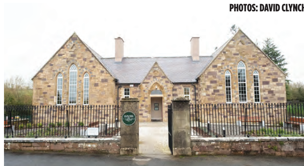
Clonea Power Community Facility.
